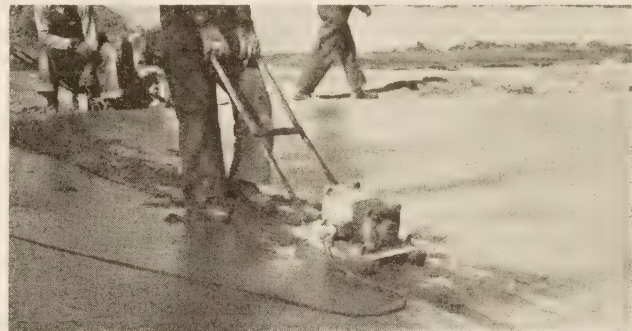
FIGURE 14.—CONCRETE FINISHING MACHINE, SHOWING PAN-TYPE VIBRATOR MOUNTED BETWEEN THE TWO SCREEDS.
